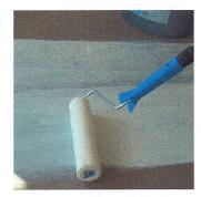
5. Apply adhesive evenly and fully to subfloor, forming a complete adhesive film. Avoid adhesive pools.
