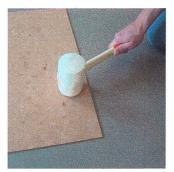
7. Lay down the cork tiles to fit and knock tightly and completely with a rubber hammer to ensure a complete bond formation.
