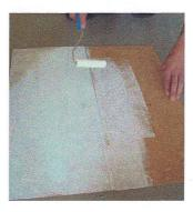
3. Apply adhesive evenly and fully to cork backing, forming a complete adhesive film. Avoid adhesive pools.
