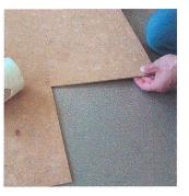
8. Lay down further cork tiles to fit and knock tightly with a rubber hammer.
